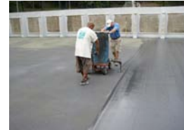
11. APPLYING ACR SEAL
