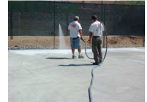
8. SPRAYING WITH POLYMER
